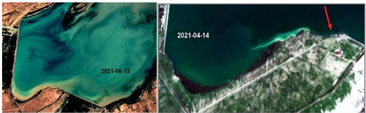
Fig Fig.3. Erosion of the south coast during strong winds (left) and the threat of outburst of the south bank of the reservoir in April 2021 (right)
