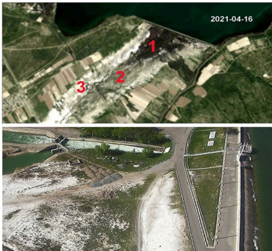
Fig. 6. Strong salinization of bog (1), meadow-bog (2) and meadow-serozem soils downstream of the Karazhantak dam (above) and the slope of the Bugun dam (below)
